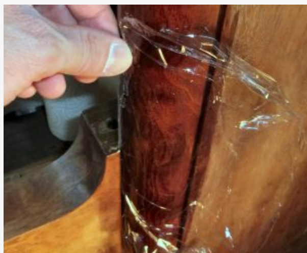
Protecting the new patch so we can test the best approach to graining.
