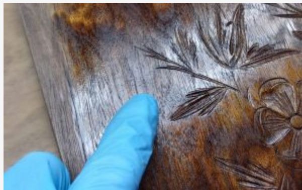
After a light sanding, the scratch is gone (a little paint thinner has been applied to highlight the wood - which would make any remaining damage more visible)
