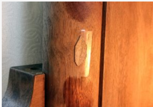
Laying out the patch
